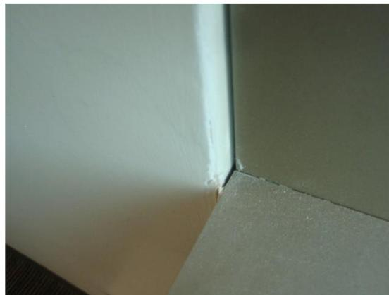
Figure 65: The gap in the same wall shown in Figure 64, where the wall meets the window
